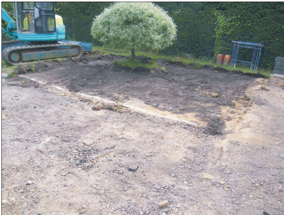
Plate 2: Site fully excavated
