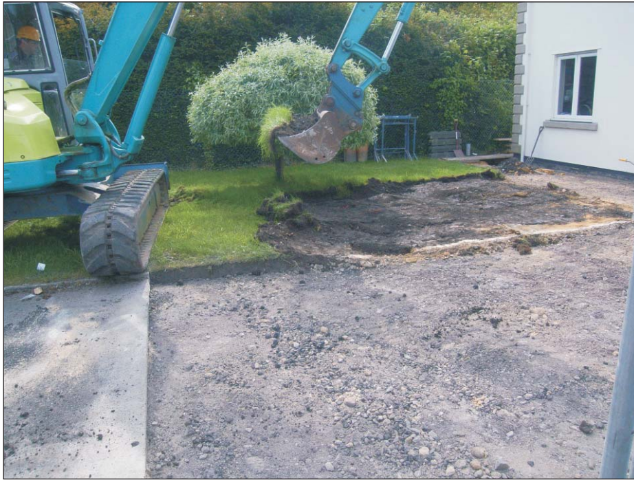
Plate 1: Excavation of site
