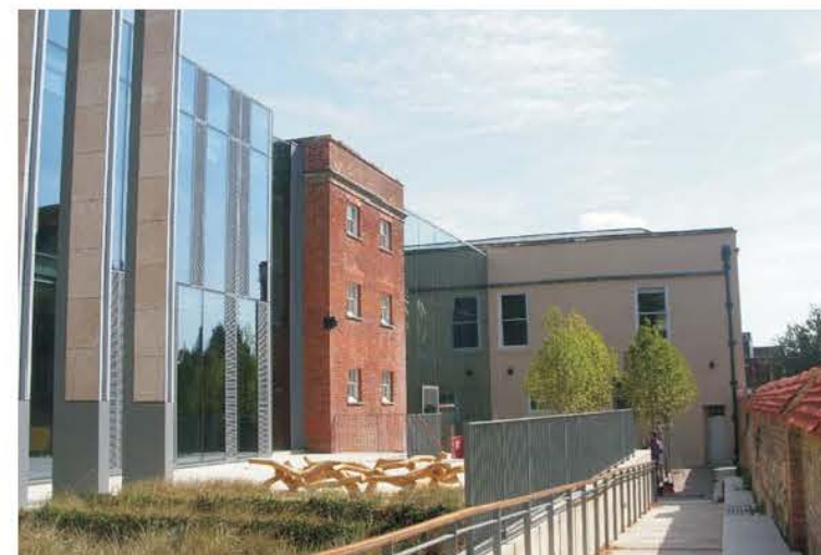
32. Unfolding view of the Long Garden with reflections of the south wing within the new glass additions.
