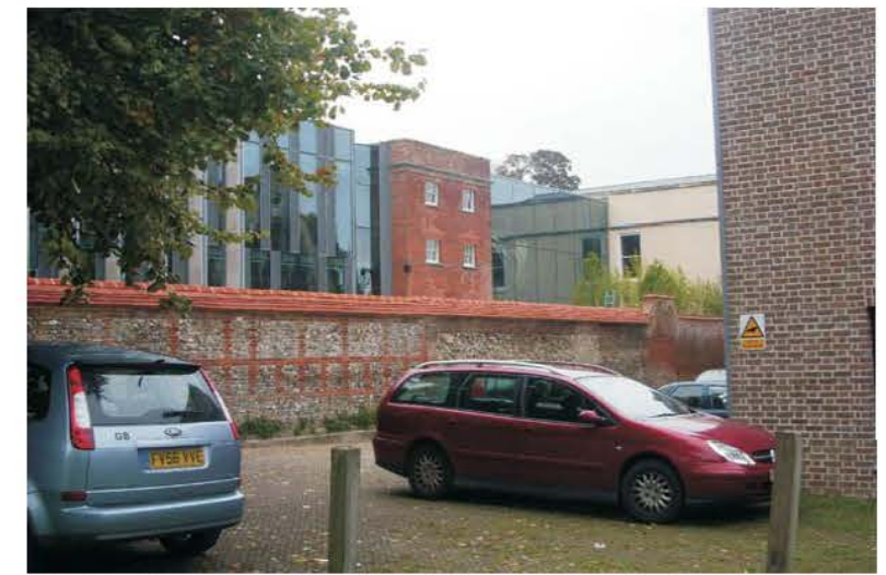
21. The modern extension, the glass additions and the south wing of Council House, as viewed from the car park of the Salisbury Arts Centre
