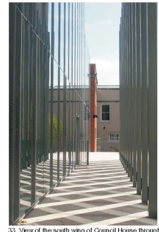
33. View of the south wing of Council House through the west colonnade of the modern extension.
