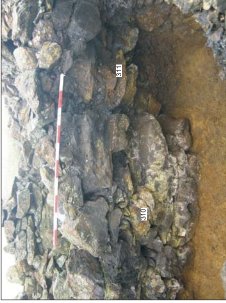
Plate 8: South-west facing elevation of wall 310 and doorway blocking wall 311 (scale 1m)
