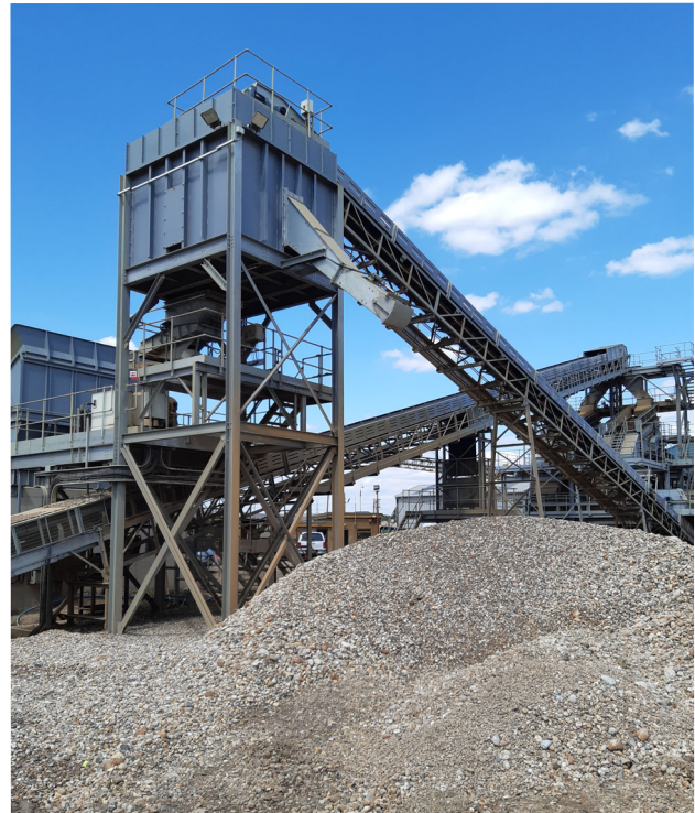
Hanson Dagenham Wharf
