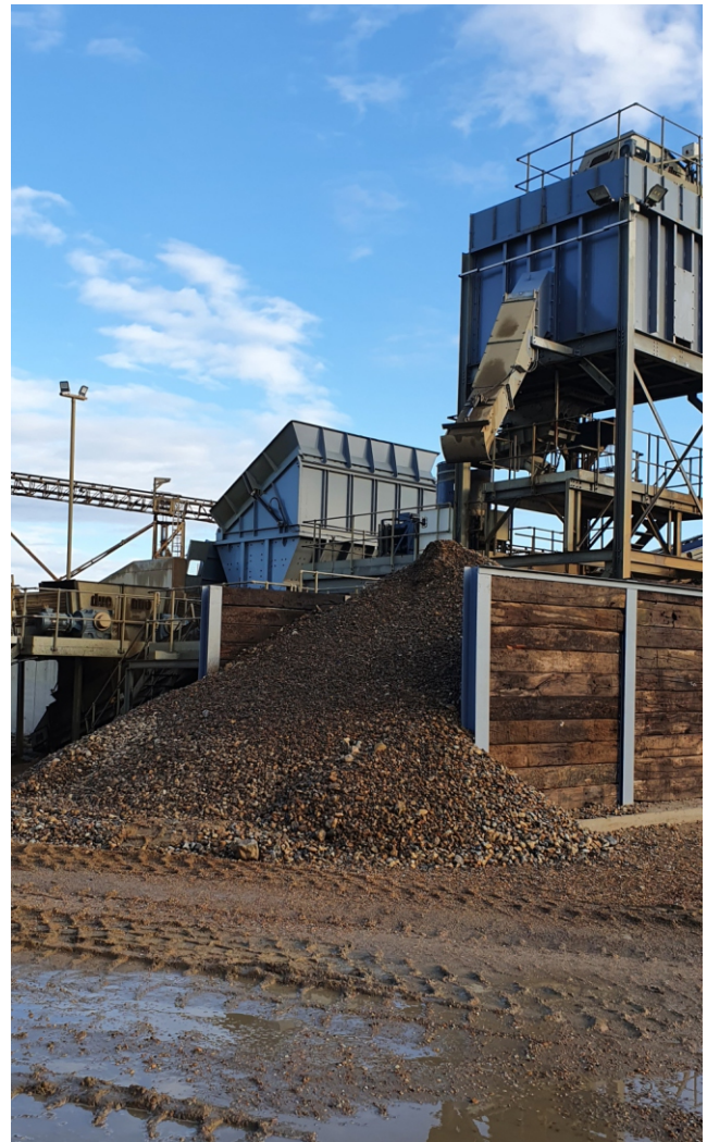
New bay at Dagenham Wharf for isolating Area 240 cargoes
